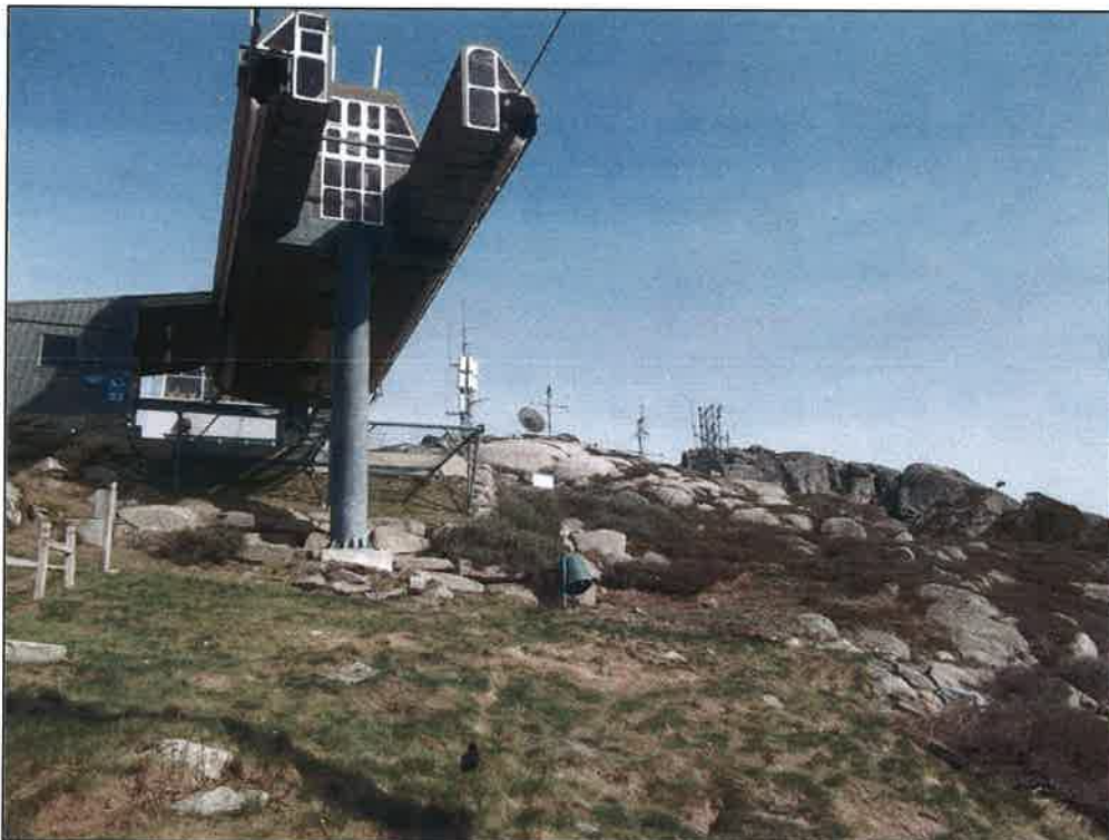
Photo 8: Eagles Nest existing facilities location looking west from top of mountain. Note the 'antenna farm presentation to visitors.
