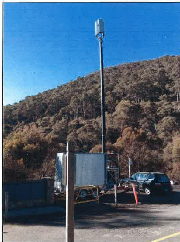
Photo 10: Temporary Cell On Wells (COW) Optus site installed for 2014 Ski Season. Note the occupying of valuable Thredbo Village real estate, visual impact, security and safety risks.
